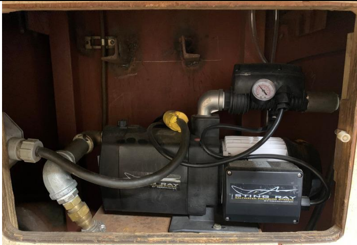
Water pressure pump
