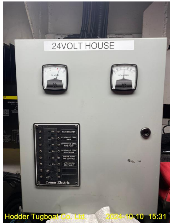
Electrical distribution panel
