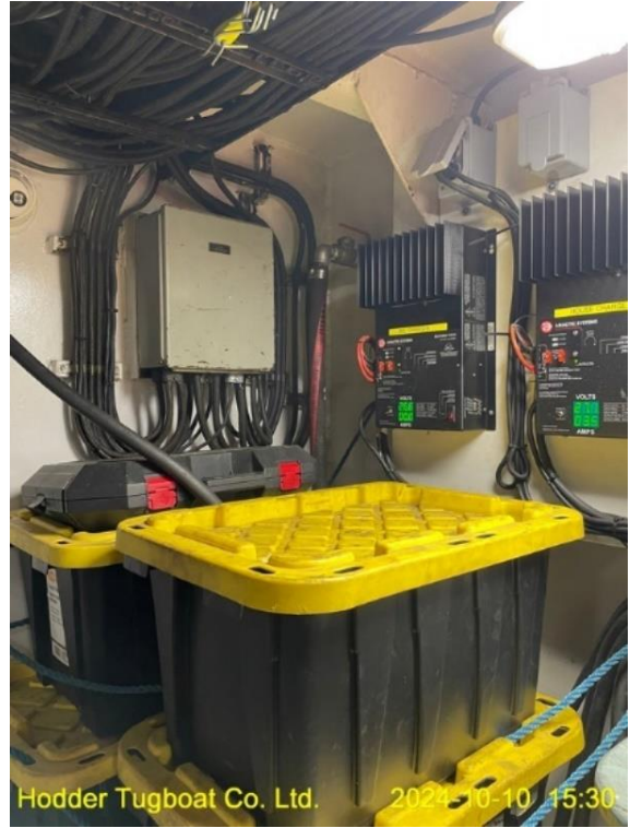
Battery charging setup and it's electrical cabling
