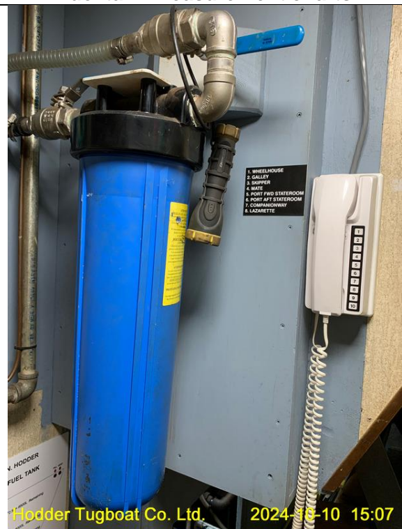
Water filtration unit and intercom phone
